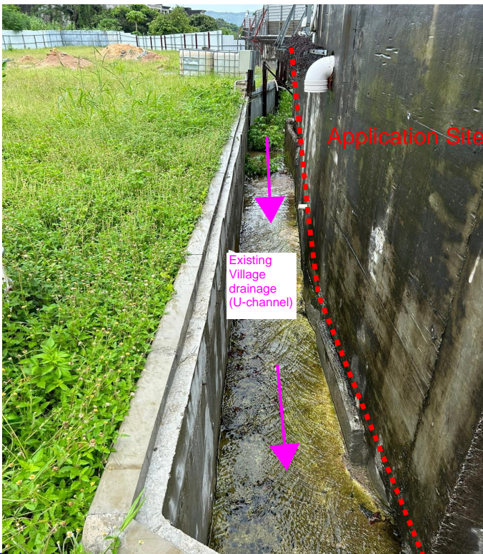
Site Photo 1 for existing village drainage
