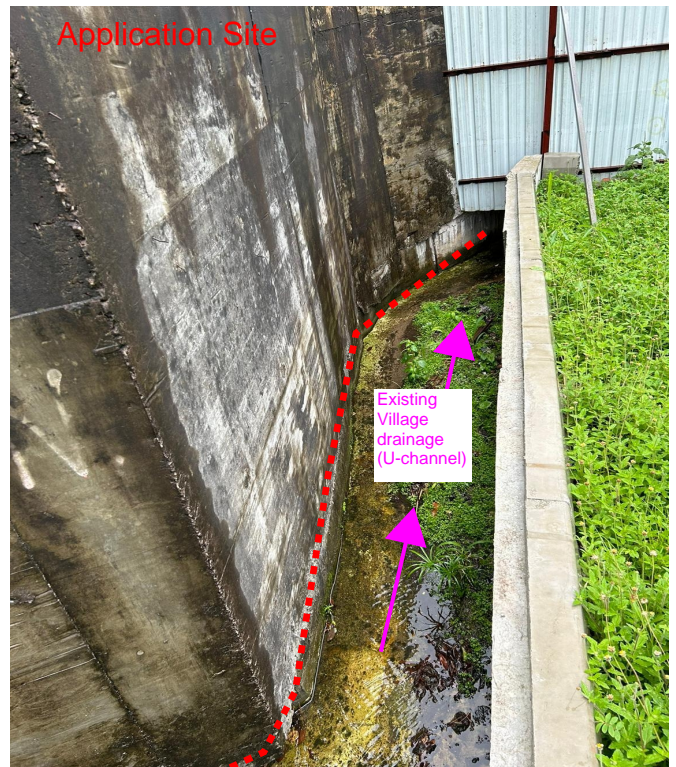
Site Photo 2 for existing village drainage
